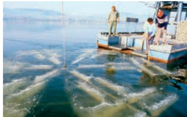
Air and, if needed, pure oxygen is introduced into the depths of the lake with diffusers
