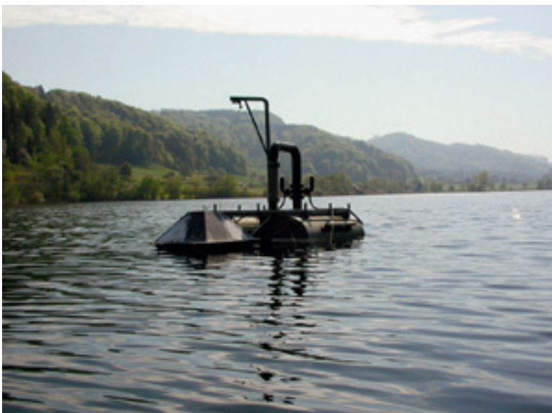
The artificial mixing system in Lake Türler leads to complete mixing and increases deep-water oxygen levels.
