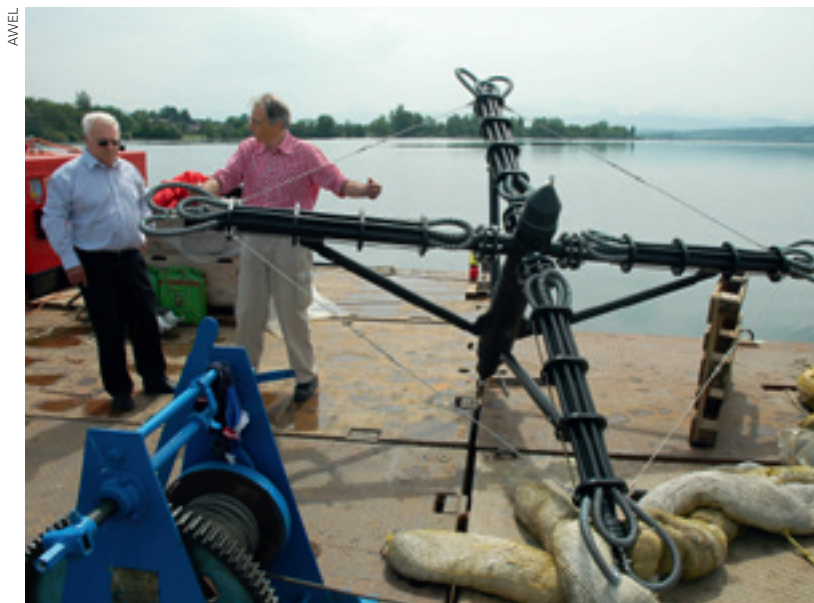
Assembly of the diffusion system which is to supply Lake Greifen with oxygen.
