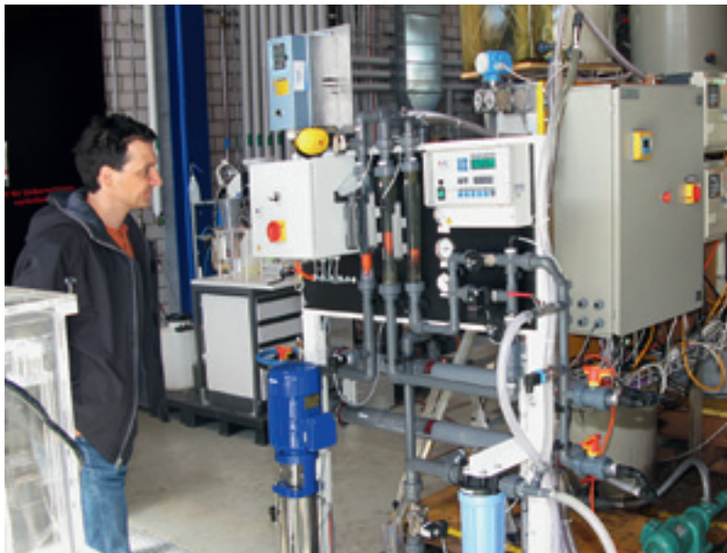
Anammox pilot reactor at the Eawag testing facility.
