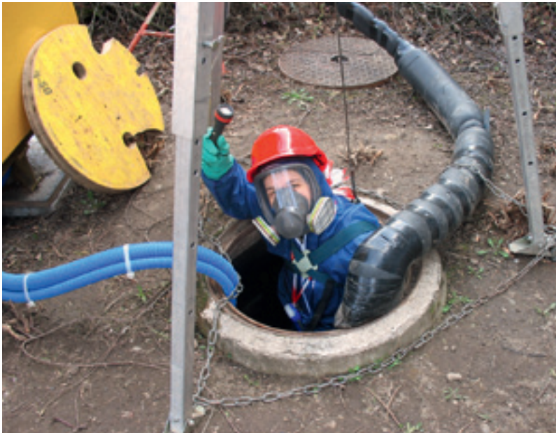
Lubomira Kovalova climbs into a sewer at the Baden Cantonal Hospital, where wastewater is collected for the pilot plant.
