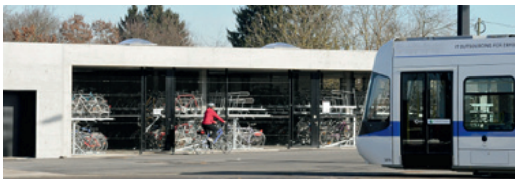
The lockable bike shelter at Stettbach station.
