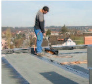
Root-resistant bitumen sheets are used to seal a flat roof which is to be extensively vegetated.
