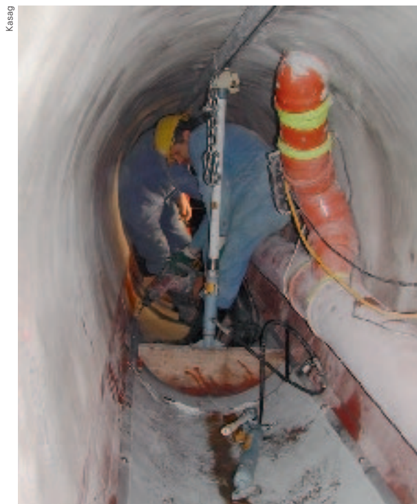
Installation of a heat exchanger in a main sewer pipe.
