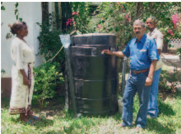
Compact biogas system for a household in Dar es Salaam (Tanzania). Although the plant (originally developed in India) is functional, there is a lack of data, e.g. on gas yield and composition. This makes it difficult to optimize the system and adapt it to local conditions in Africa.
