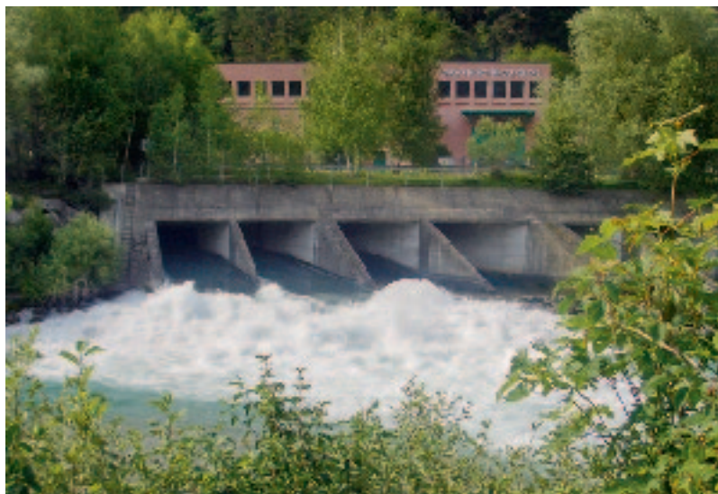
Discharge of water below a hydropower plant on the Anterior Rhine.
