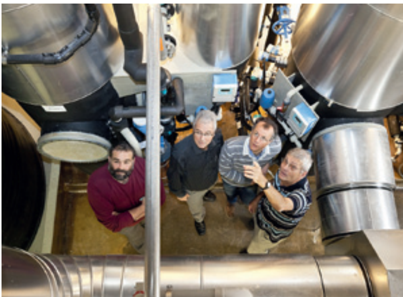
Hansruedi Siegrist and Marc Böhler of Eawag with Christoph Liebi and Pascal Stutz of the Kloten/Opfikon WWTP (from right to left). Behind them are the three reactors where the stripping process takes place.
