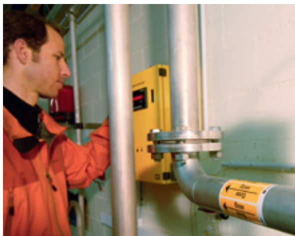
Additional treatment with ozone gas can effectively eliminate many micropollutants from wastewater.
