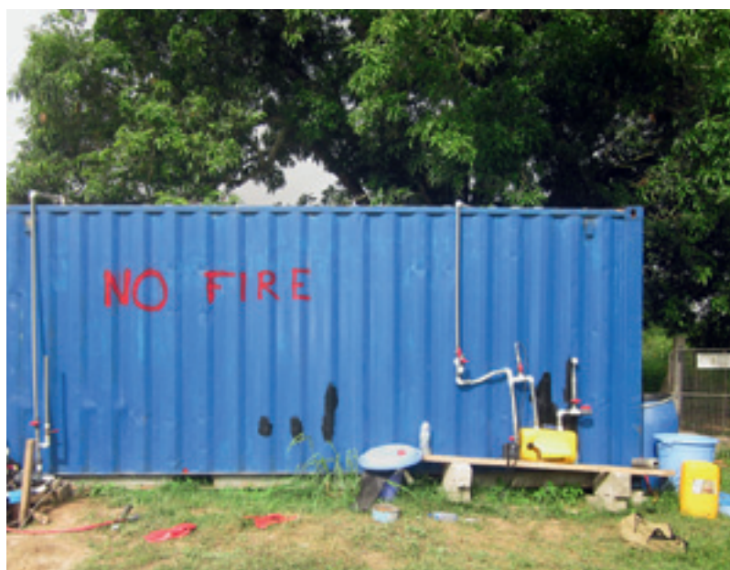
Functional, but not economically viable: a biogas plant in Ghana.
