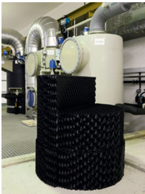
To increase the surface area, the reactor columns are fitted with plastic packing elements arranged in a honeycomb structure.
