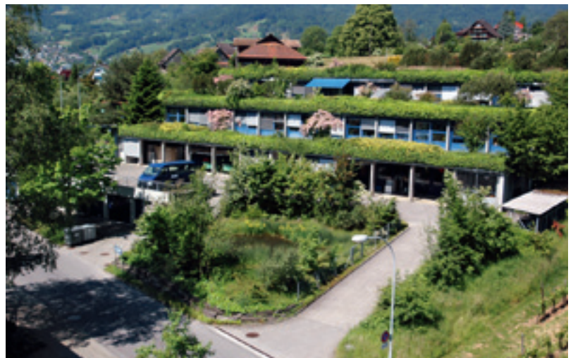
Renovation work has begun on the 1970s-era terraced facility at Eawag's Kastanienbaum site.
