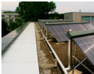
Photovoltaic solar panels are one of the renewable energy sources used by Eawag.
