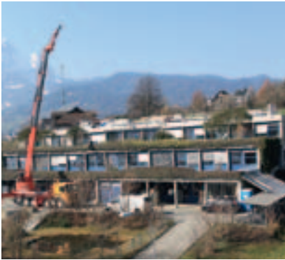
Renovation of the laboratory building at the Kastanienbaum site was completed in 2012.
