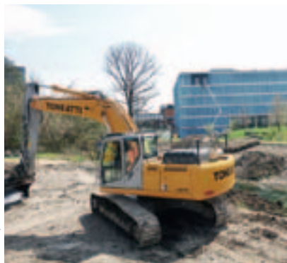
Work has begun on restoring the degraded Chriesbach stream.
