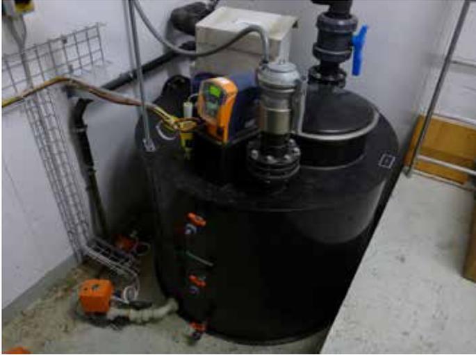
**Figure 6:** The urine storage tanks at Eawag each contain 1 000 L urine to attenuate daily and weekly fluctuations. The urine dosage pump (orange/blue) is installed on the tank.
