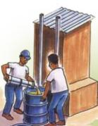
Urine from the urine diverting toilets and waterless urinals is collected in small tanks attached to the toilet foundation walls.
