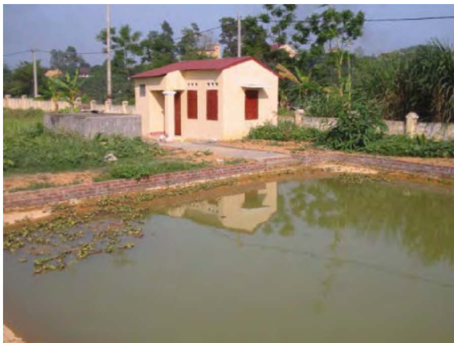
Figure 9.7 Basic lagoon system at a hospital
