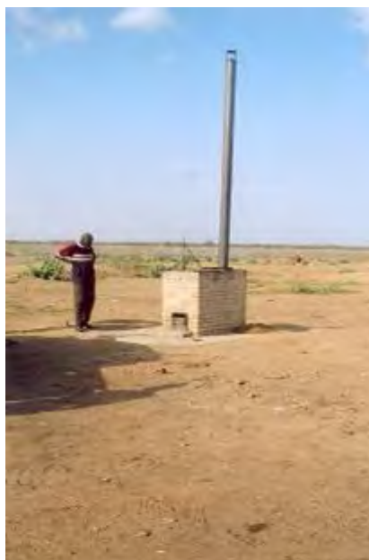
Figure 14.3 Double-chamber incinerator in a health-care centre dumping site
