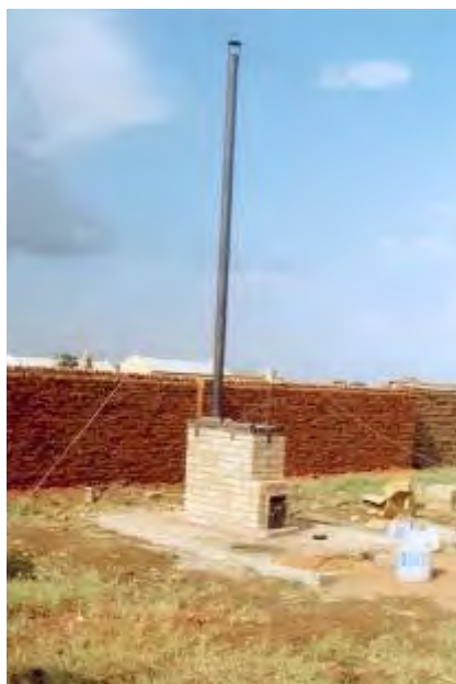
Figure 14.3 Double-chamber incinerator in a health-care centre dumping site
