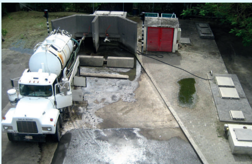
Figure 9.10 Faecal sludge discharge at Illidge Road wastewater treatment plant at the buffer tank.
