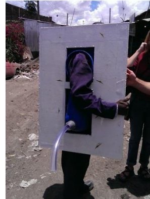
Pre-fab urine-diverting squatting pan ready for installation (right)
