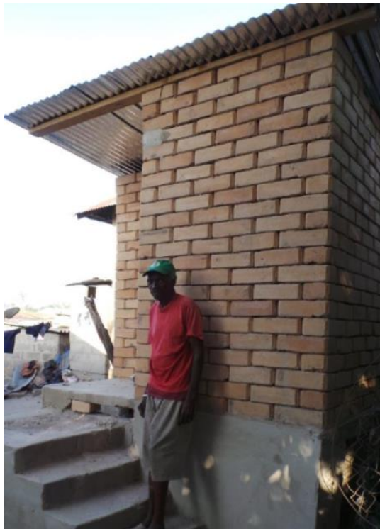
Figure 5-4: Soil cement blocks used in Dar es Salaam, Tanzania. © Centre for Community Initiatives.
