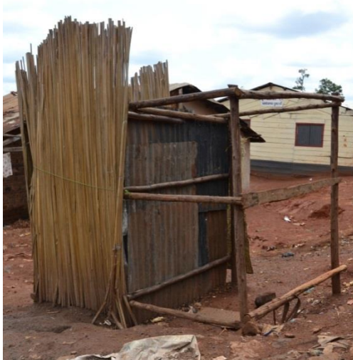
Figure 2: Sub-standard pit latrine in Kampala, Uganda.
