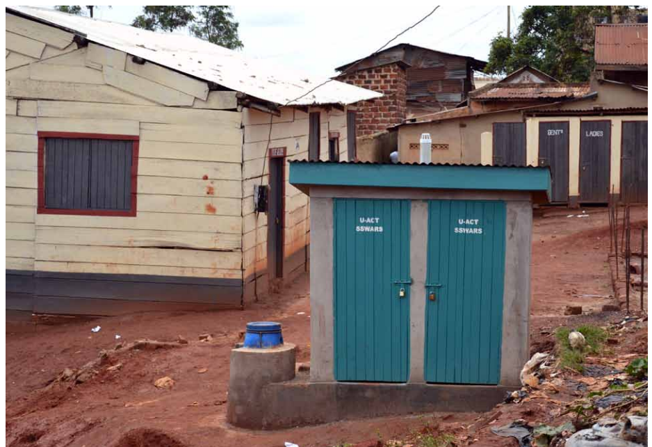
Photo 1: New double stance shared toilet facilities built in 2012 using targeted subsidies.
