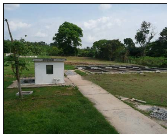
Figure 4: Project site at the KNUST sewage treatment site
