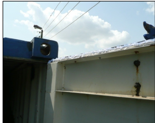
Figure 27: Silicon sealant applied to the rubber sealing of the door
