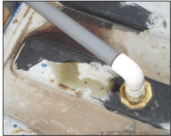
Figure 29: PVC pipe connected at container top
