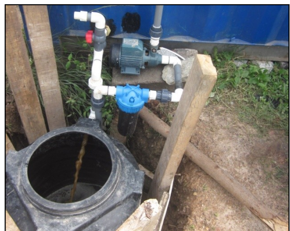
Figure 33: Percolate storage tank
