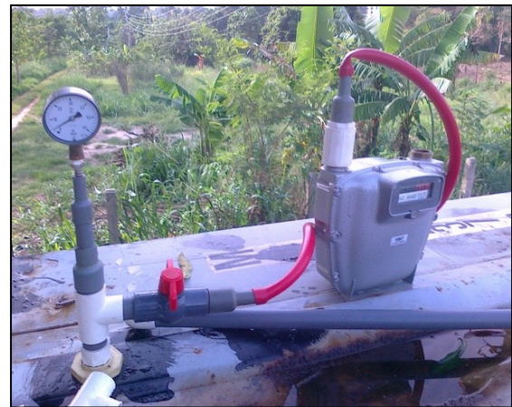
Figure 10: Gas meter test to estimate amount of leakage
