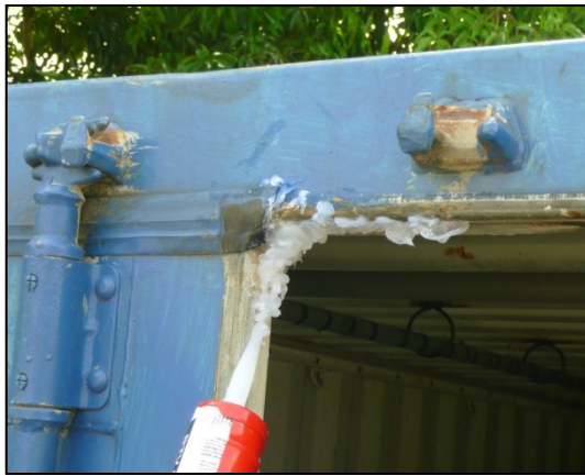
Figure 26: Adding silicon sealant before closing the door
