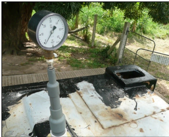
Figure 9: Pressure meter test to find the maximum pressure build up.
