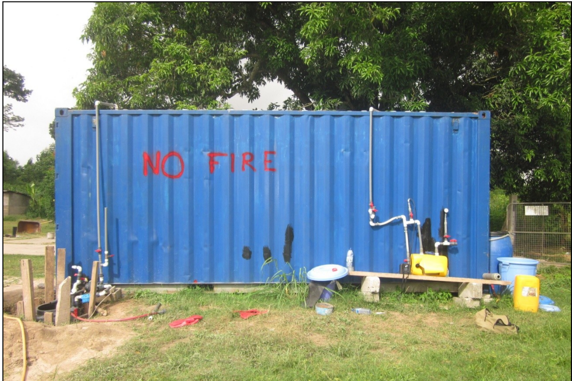
Figure 22: Side view of the shipping container
