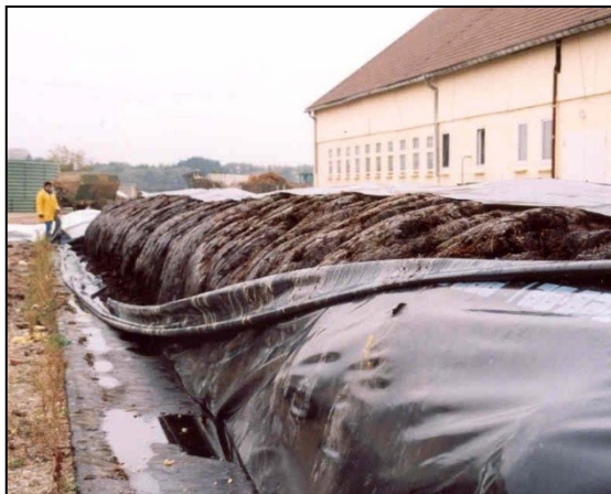
Figure 18: Polyfoil digester in Germany. Being cut open to remove the digestate (LfULG 2002).
