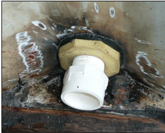
Figure 28: PVC fitting for 1'' pipe connection
