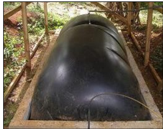
Figure 19: Polyfoil wet digester in Costa Rica. Gas storage directly in the poly bag (RCR 2006).
