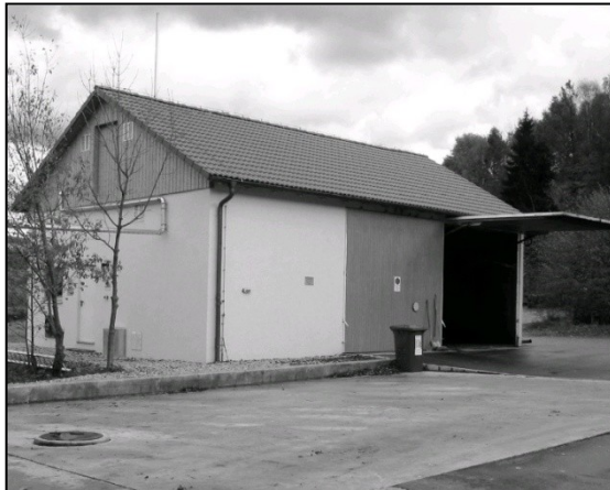
Figure 20: German garage digester built from bricks and concrete with a custom made air tight door (Gronauer and Aschmann 2003).
