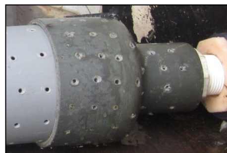
Figure 14: 3" PVC filter pipe. Prevents coarse particles from getting into the external part of the percolation system.
