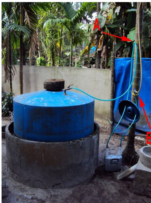
Figure 17: Connected gas meter. The fixation (A) enables the gasholder to move freely. The “three ways” installed at the point B enables to carry out \text{CO}_2 measurements.
