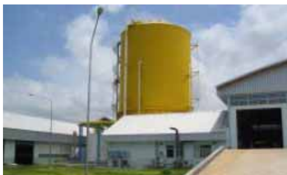
Picture 28 and 29: Rayong Municipality Co-Generation Plant: On the left-side the digester, and on the right side the gas storage.
