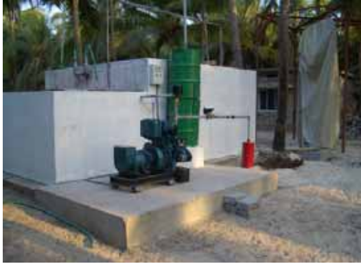
Pictures 22 and 23: Biogas plant in Kavaratti, India treating residues from fish processing and small amounts of kitchen waste
