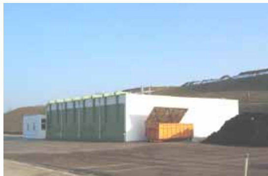
Picture 31: Bekon GmbH biogas plant in Fröttmanning (Munich), Germany. The plant consists of four parallel operating batch digestion reactors. Feedstock material is mainly biodegradable municipal waste. (Source: Bekon GmbH)
