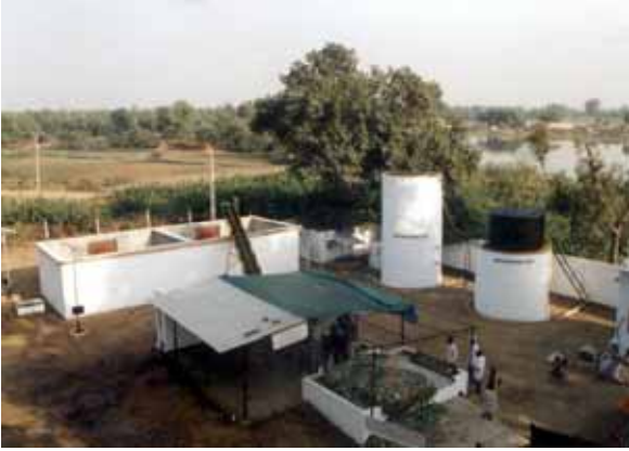
Picture 14: SPRERI biogas plant in Anand, India converting vegetable market waste into biogas and compost. Plant commissioning was in 2004, but until now the plant is operating under its design capacity (Source: SPRERI).
