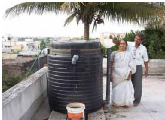
Picture 11: ARTI biogas plant for treatment of kitchen waste at household level.
