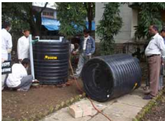
Picture 10: Construction of an ARTI compact biogas plant.
