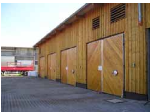
Picture 30: Bioferm GmbH biogas plant in Iffezheim, Germany. The plant consists of four parallel operating batch digestion reactors. Feedstock material is renewable raw material, such as maize. (Source: Sandec).
