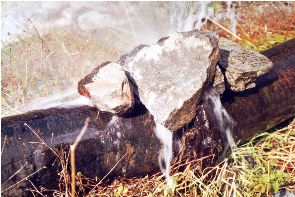
Picture 2: Leaking pipes are often repaired with wooden sticks, cotton rags or stones. (Picture: Bettina Sterkele)
