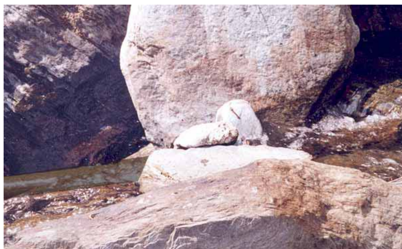
Picture 1: Water source intake structure. The intake pipe (enhanced in colour on the left had side) is fixed by stones into the river pool (centre)
