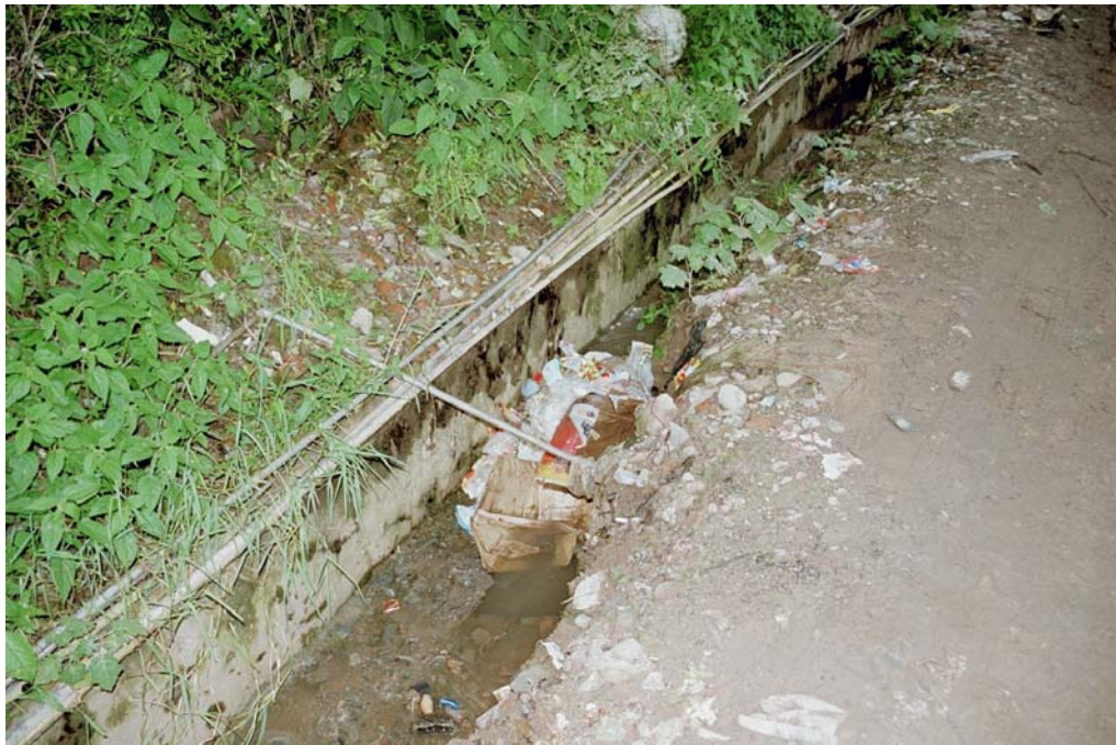
Picture 4: Open drain in McLeod Ganj in dry season. The drain is in a relatively good condition but the waste lying inside might block it in rainy season and the water pipes though relatively high might be flooded. (Picture: Gabriela Friedl)
