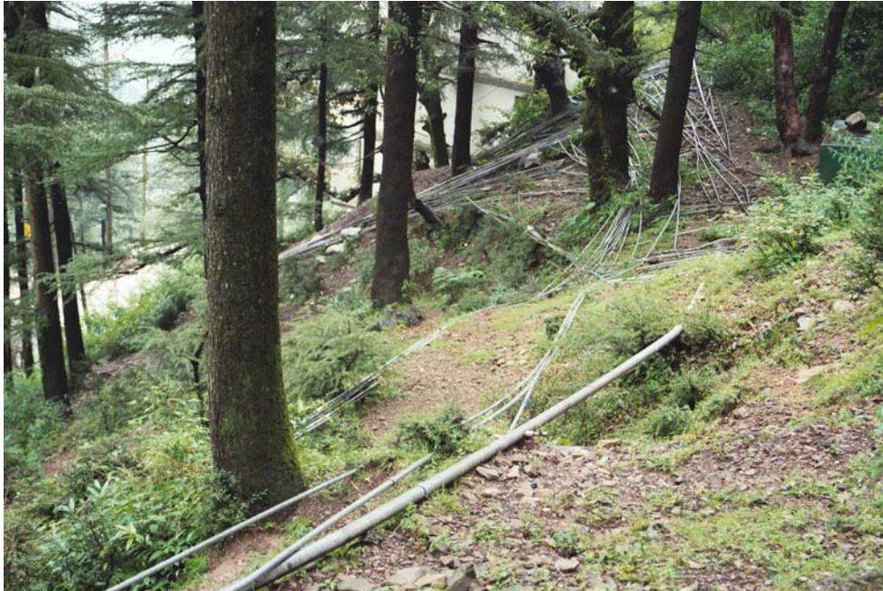
Picture 3: Many household pipes are going parallel as they have to, or prefer to connect on a high level of the main pipe. (Photo: Gabriela Friedl)
