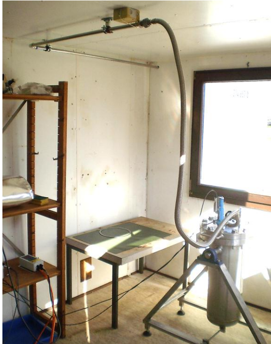
General view with stainless steel pipe for exhaustion of steam from overpressure valve
