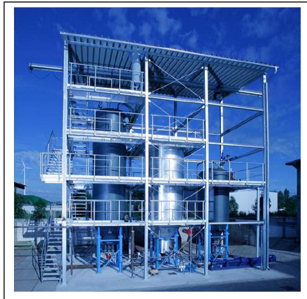
Figure 11: Picture of the HTC plant in Karlsruhe (Source: AVA-CO2 leaflet)
