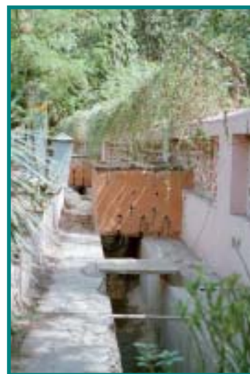
Compost Bins on a Drain
