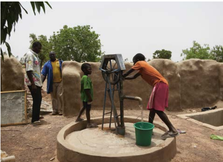
Photo 1: Upgraded well with rope pump on premises.
