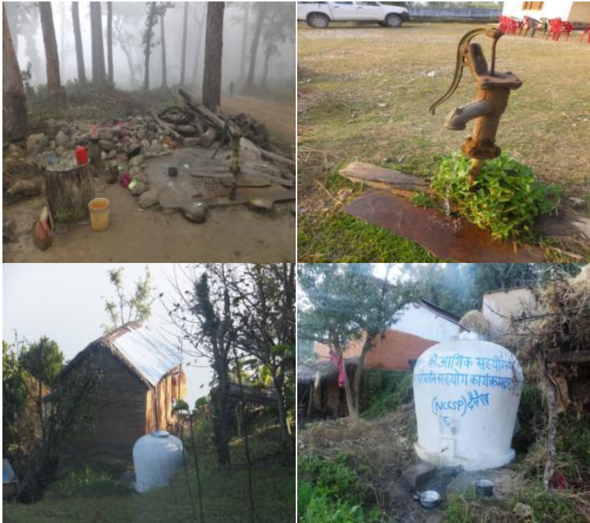
Figure F.2 handpump (tubewell) in Kailali (top); rainwater harvesting in Dailekh (bottom)
