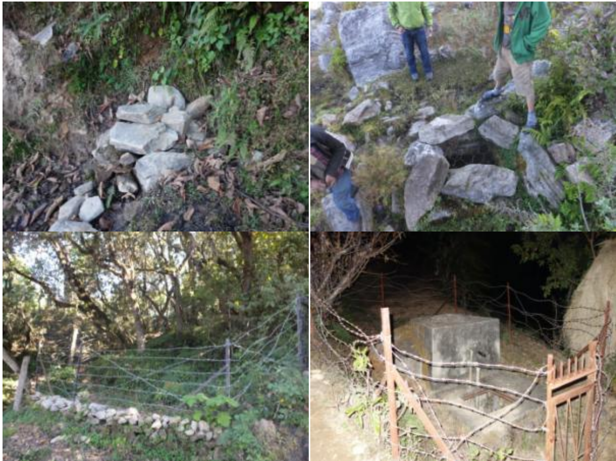
Figure E.2 Source protection: (top right) just cover by stone in Acham; (top left) stone + wire but still accessible by animal and human in Acham; (bottom left) protected by wire in Acham; (bottom right) protected by concrete and wire
