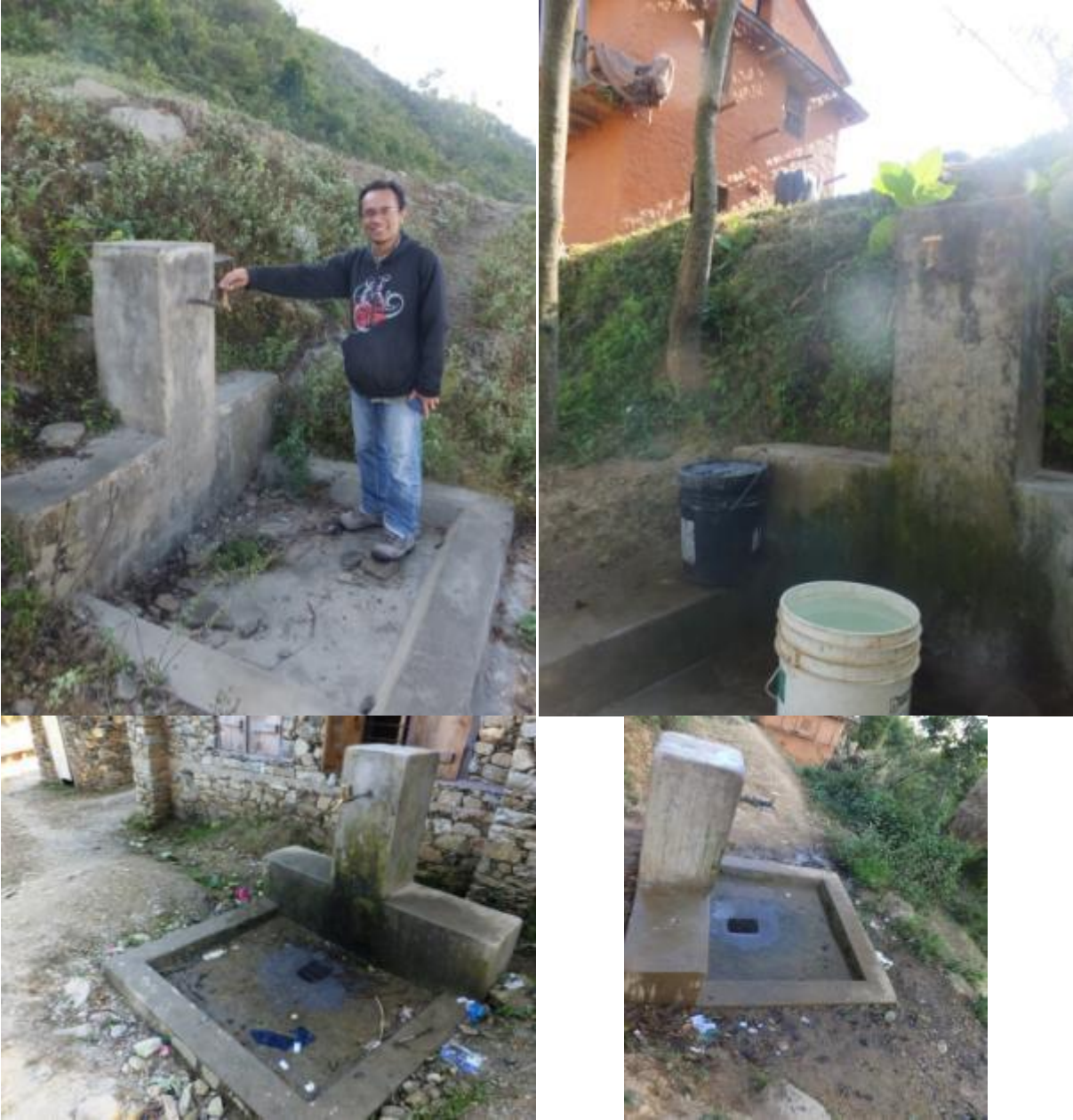
Figure F.1 public tap: (left) not working, location; (right) working; (bottom) dirty environment around tap; all pictures was taken from Dailekh
