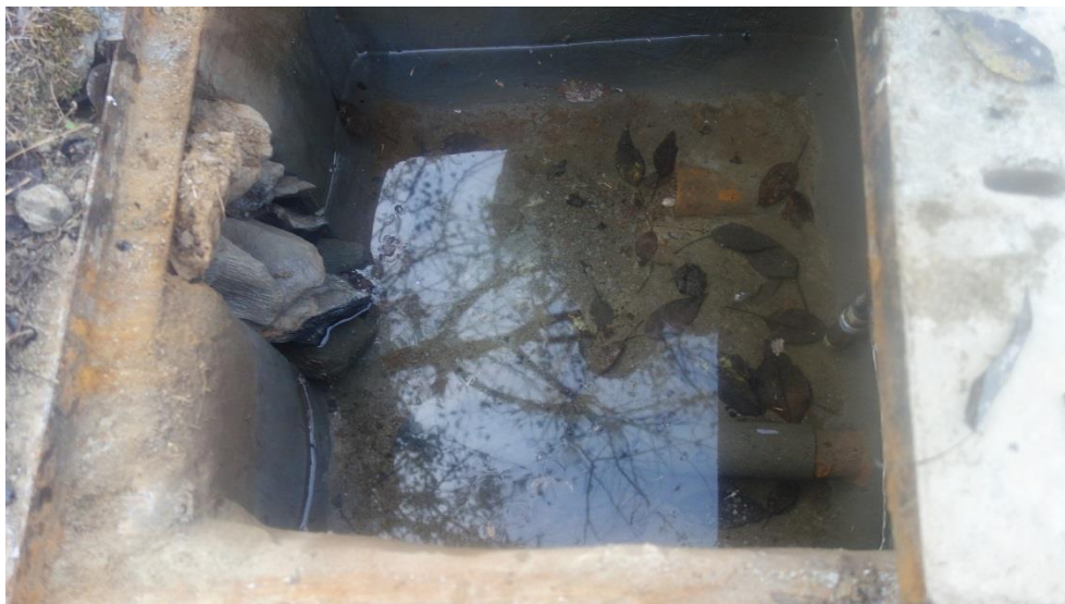
Figure 42 Intake of iPWS IV
