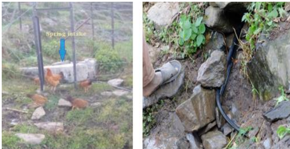
Figure 20 Spring of iPWS II and leaking pipe
