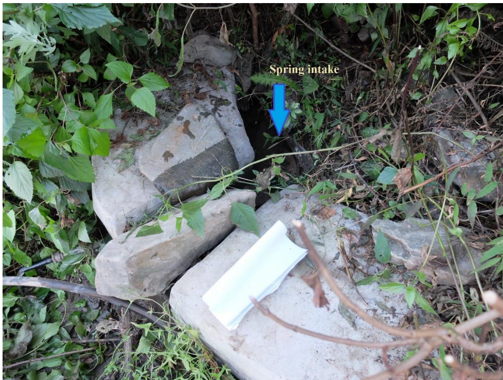
Figure 31 Shows the intake of the spring and pipe connecting the outlet to reservoir
