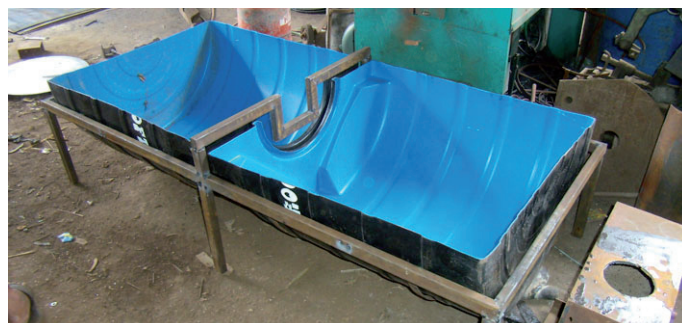
Figure 11: The reactor frame under construction.
