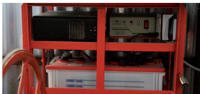
Figure 14: Battery and charger are locked up in metal cage.
