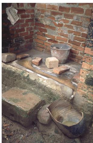
Double-pit latrine with urine diversion (Viet Tri, Vietnam): latrine floor with openings to the two chambers for faeces, a urine diversion channel and a urine pot.
