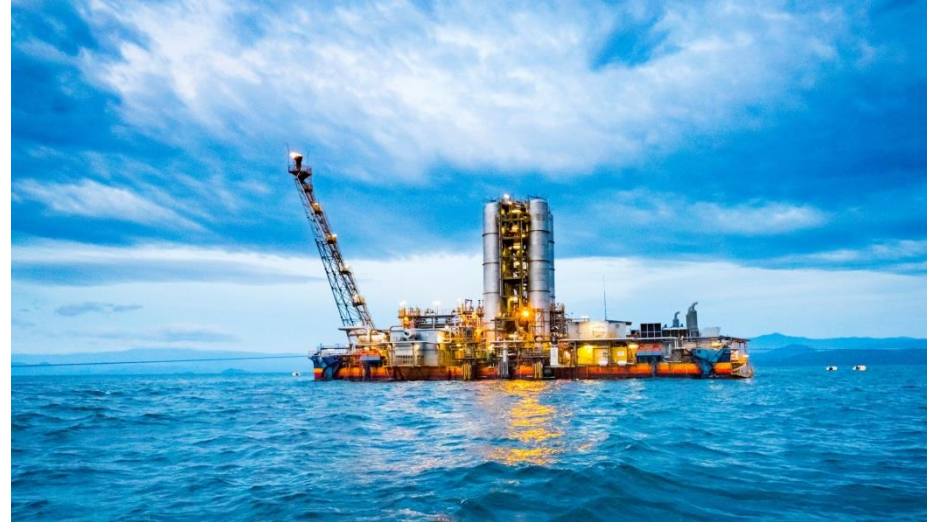
ContourGlobal KivuWatt Anlage (25 MW)
