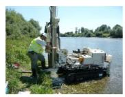
Installation of an observation well (piezometers) on a restored section of the Thur, using a Geoprobe direct-push system.
