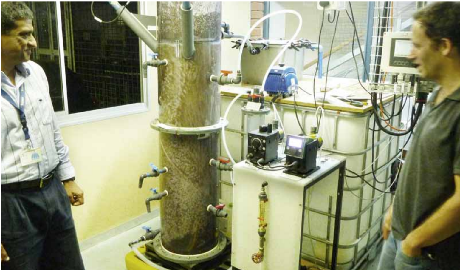
Fig. 6: Pilot plant at the Durban water utility's customer care centre.
