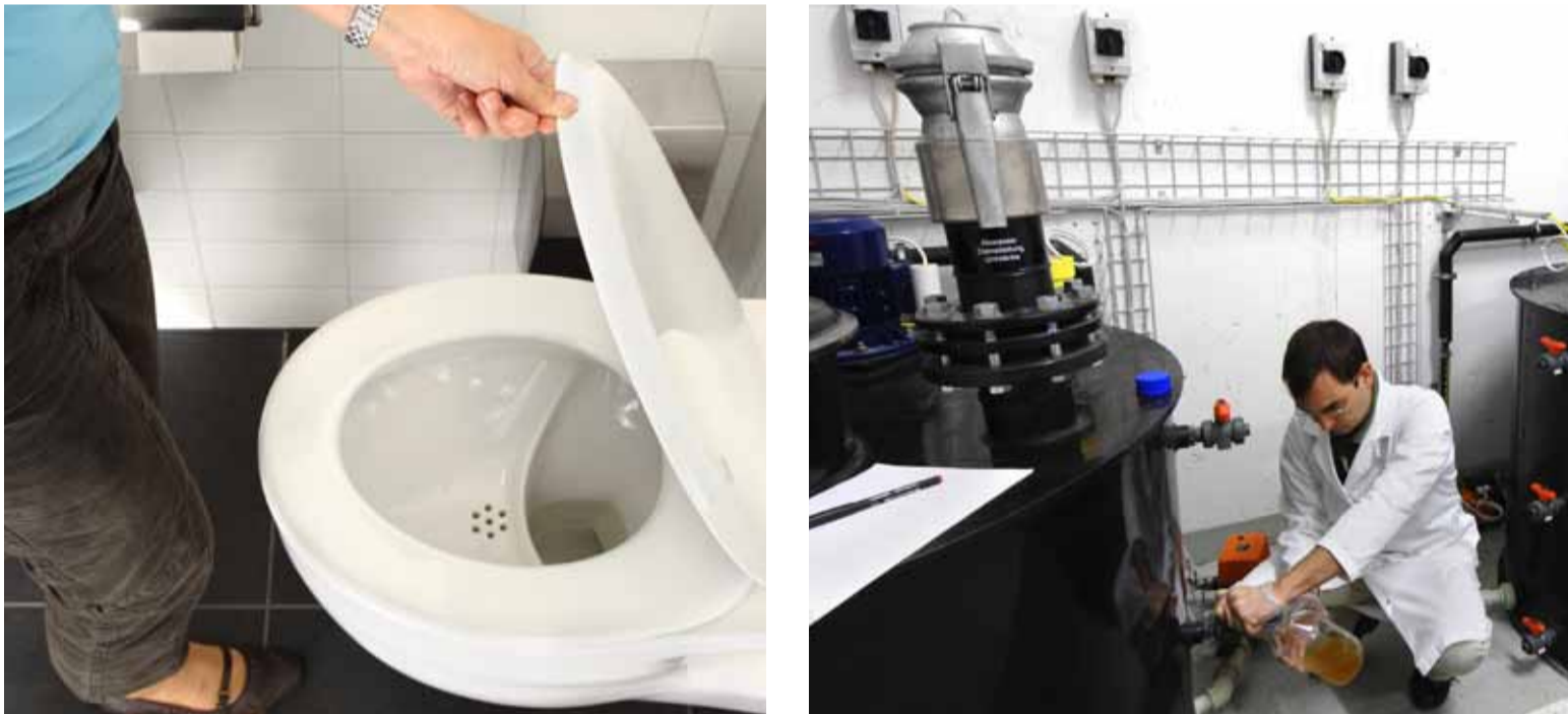
Fig. 3: Diversion toilet and separate tanks for urine storage at Eawag headquarters (Forum Chriesbach).
