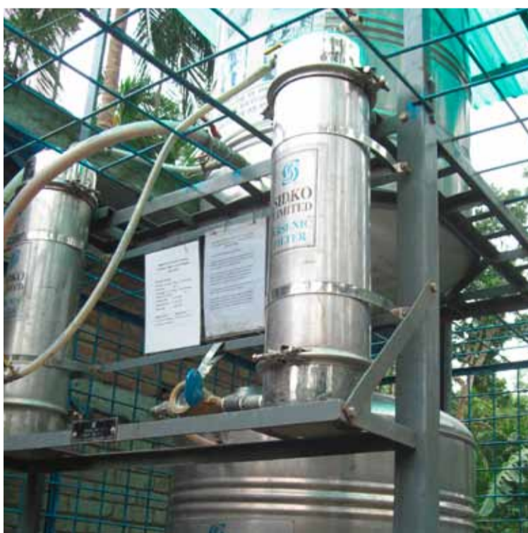
Fig. 5: A community arsenic removal filter installed in Bangladesh and a household bone char filter used to remove excess fluoride in Ethiopia.
