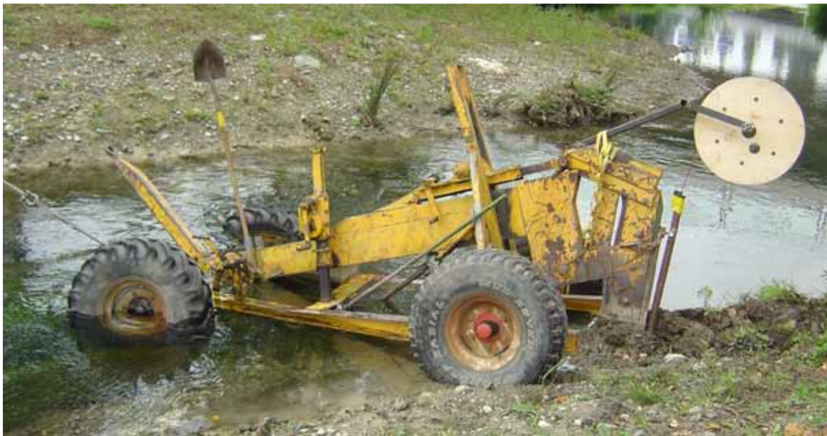
Fig. 2: Plough specially designed to install fibre-optic cable in the streambed.
