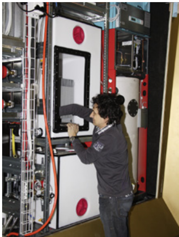
Left: A compact treatment system is installed above the grey water tank in the equipment compartment of “Self”. Centre: Membrane module for preparation of drinking water from roof rainwater. Right: Membrane module for recycling of grey water.
