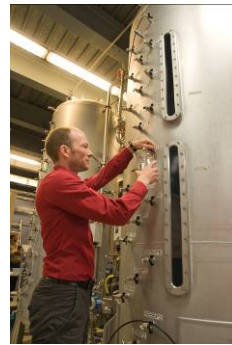
Collection of water samples from the activated carbon filter at the research and pilot plant in the Lengg lake water facility of Zurich Waterworks (WVZ)
