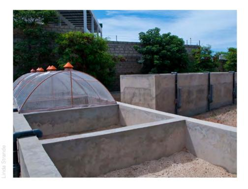
Fig. 4: Pilot-scale drying beds were used to investigate innovations to increase drying of faecal sludge.
