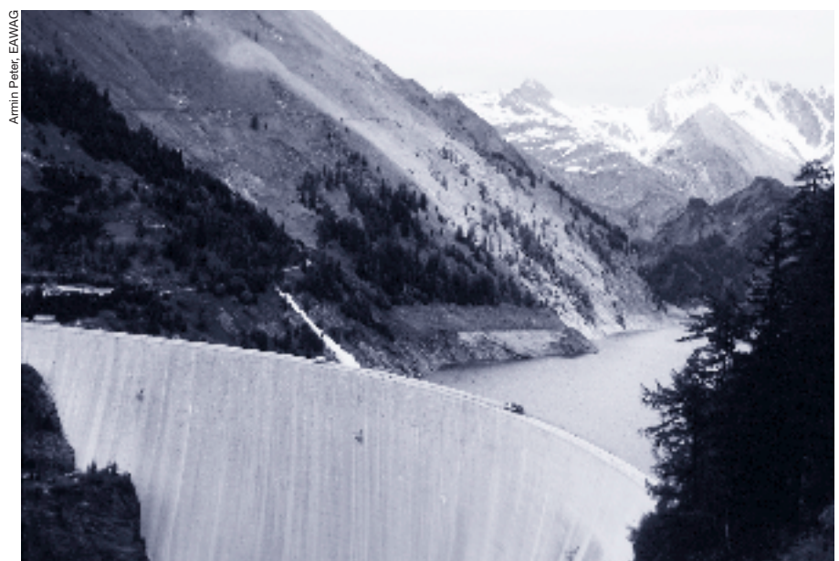
Fig. 2: The Luzzone storage reservoir in Canton Ticino. Location of the EAWAG case study “Green Electricity”.
