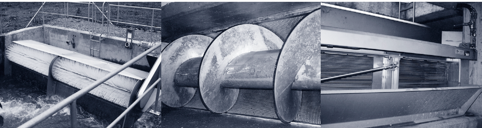
Possible remedies (from left to right): rotating brush – sieve with cleaning spiral blades – screen – underground combined sewage overflow tank – above ground combined sewage overflow tank, integrated into the landscape (bottom).
