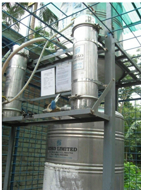
Fig. 7.3 SIDKO community arsenic removal filter installed in Bangladesh
