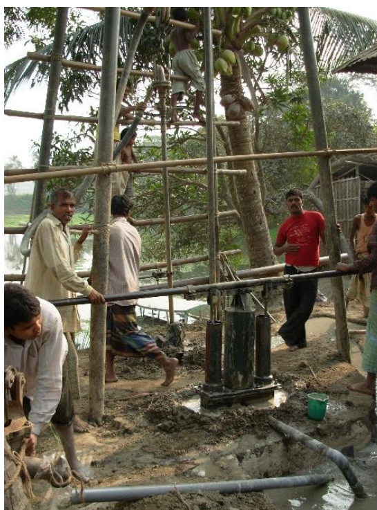
Fig. 9.6 Drilling a deep tubewell
