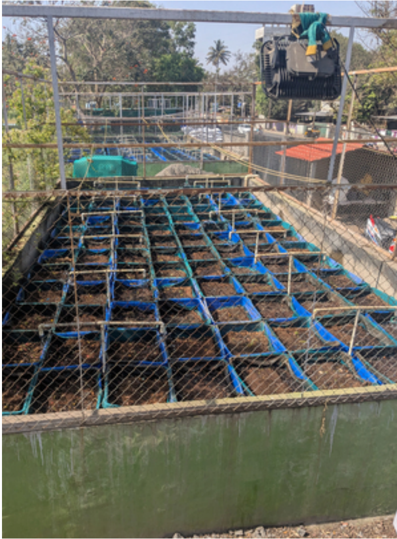
Vermifilter-installation in Pune, Indien (Foto: Kayla Coppens, Eawag).
