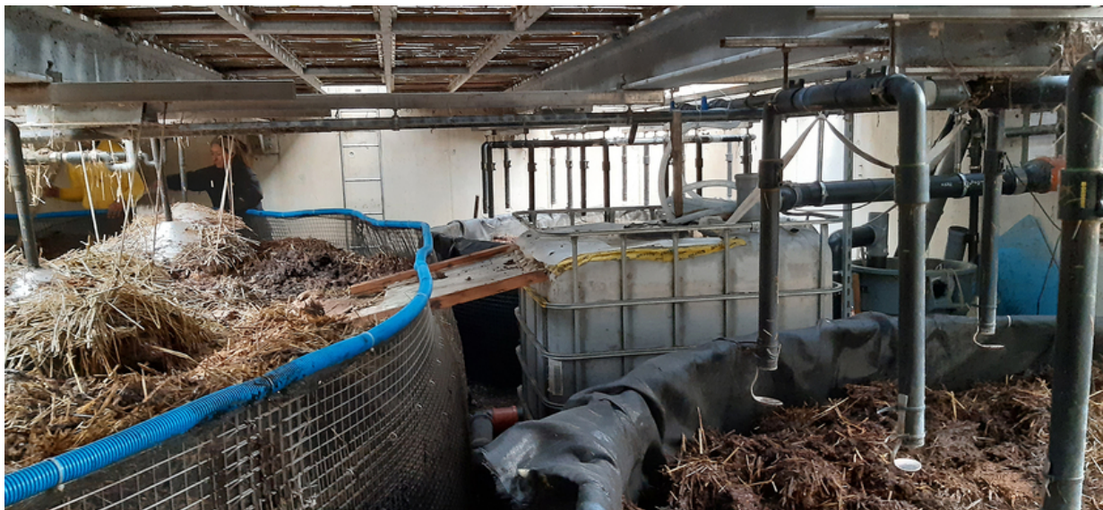
Vermifilter setup at the housing cooperative Equilibre in Geneva (Photo: Eawag, Kayla Coppens).
