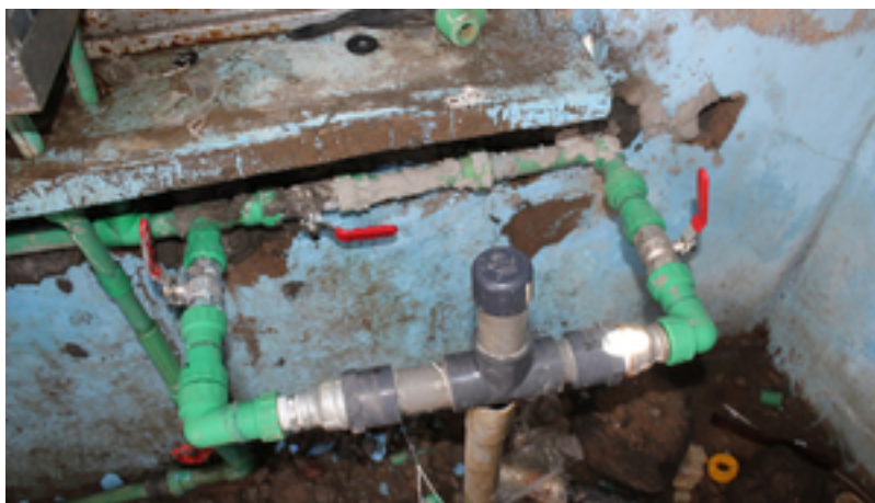
Passive, locally manufactured chlorination system installed in a water kiosk in Kenya. (Photo: Lisa Appavou)
