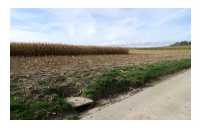
A hydraulic shortcut: water from the field and country lane is transported directly into the nearest body of water by inlet shafts such as this.
