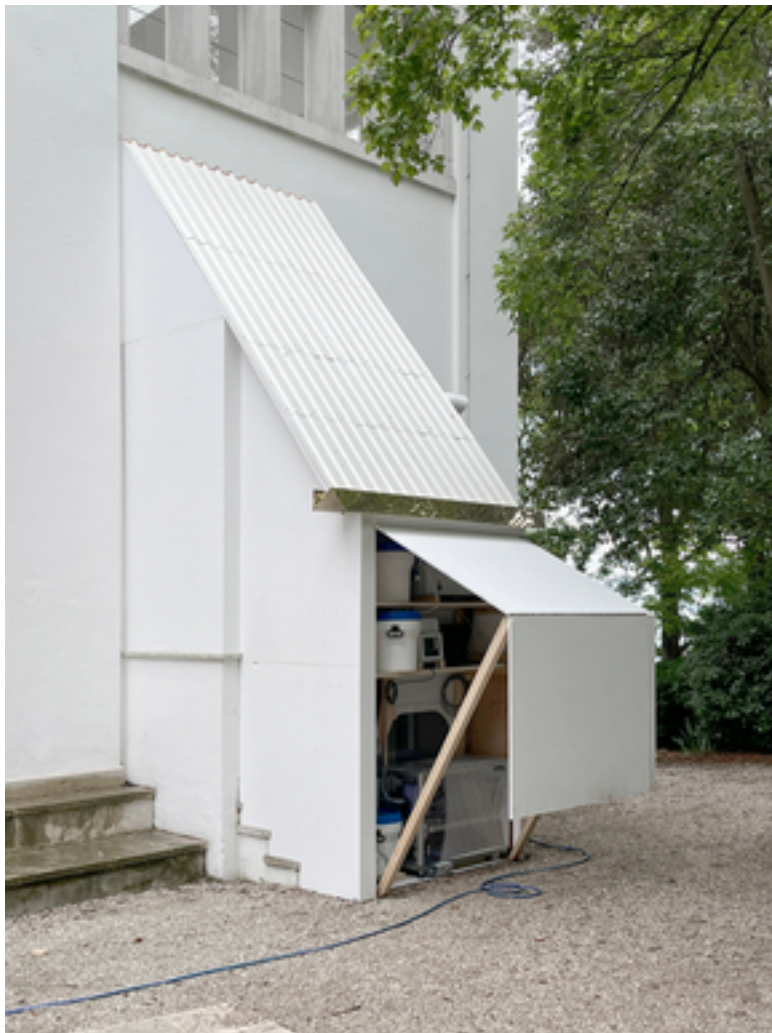
The Nutrient Harvester extracts around 1 kilogram of dry fertiliser from 30 litres of urine. (Photo: ARCH+ SUMMACUMFEMMER BÜRO JULIANE GREB)
