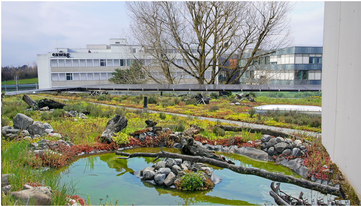
Biotope, water retention and energy storage in one: pilot plant on the roof of Eawag (Photo: Eawag).
