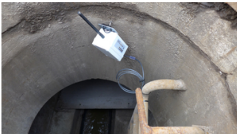
Level sensor with wireless transmission in a sewer (Photo: Frank Blumensaat, Eawag)
