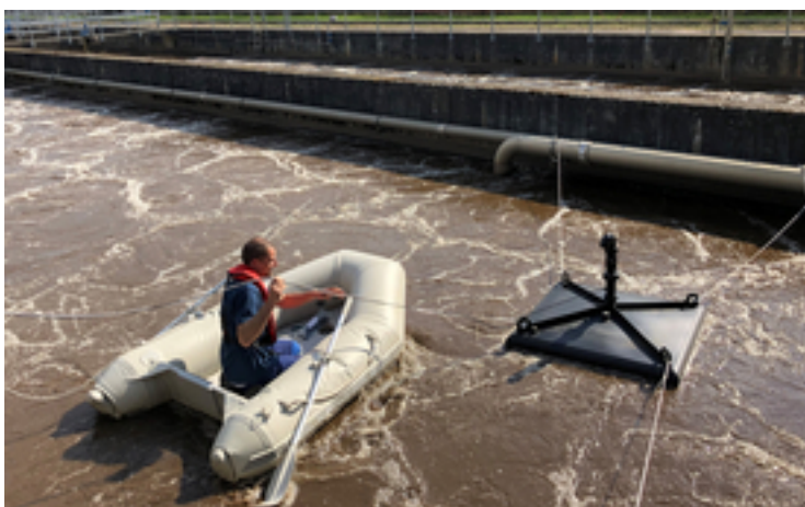
Eawag researcher Wenzel Gruber undertaking some maintenance work on the measurement system at the Moossee Urtenenbach WTP. (Photo: Andrin Moosmann)
