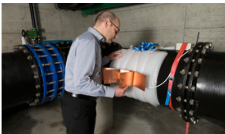
From the difference in temperature – here at the Winterthur municipal utilities between a cold water main and the surrounding environment – the energy needed for the sensor and data transmission is obtained (Foto: Patrick Cipriani / ZHAW)
