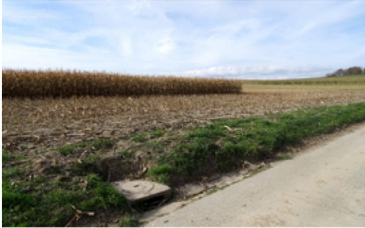
A hydraulic shortcut: water from the field and country lane is transported directly into the nearest body of water by inlet shafts such as this. (Photo: Urs Schönenberger, Eawag)
