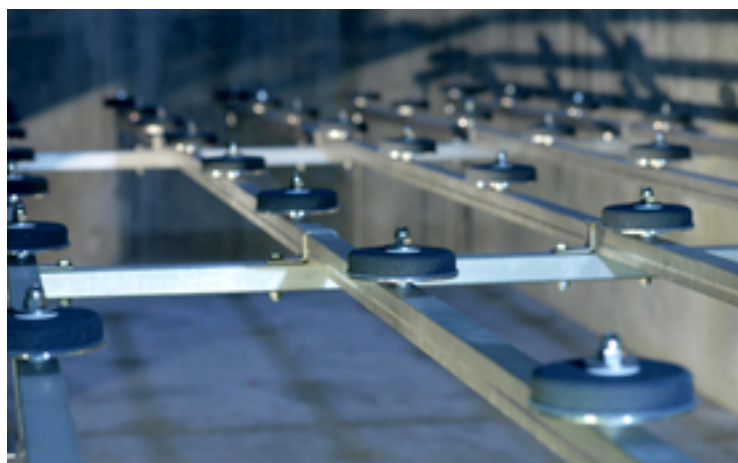
Ozonation is a proven method for removing trace substances from water. In the picture: Ozone diffusers at the Neugut WWTP in Dübendorf. (Photo: Aldo Todaro, Eawag)
