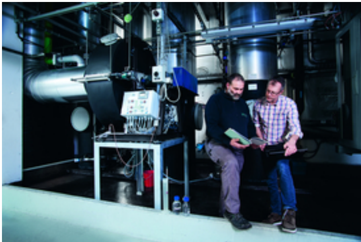
Air-stripping installation for nitrogen recovery at the Opfikon wastewater treatment plant. Photos: Eawag, Peter Schönenberger (left), Eawag, Aldo Todaro (right)
