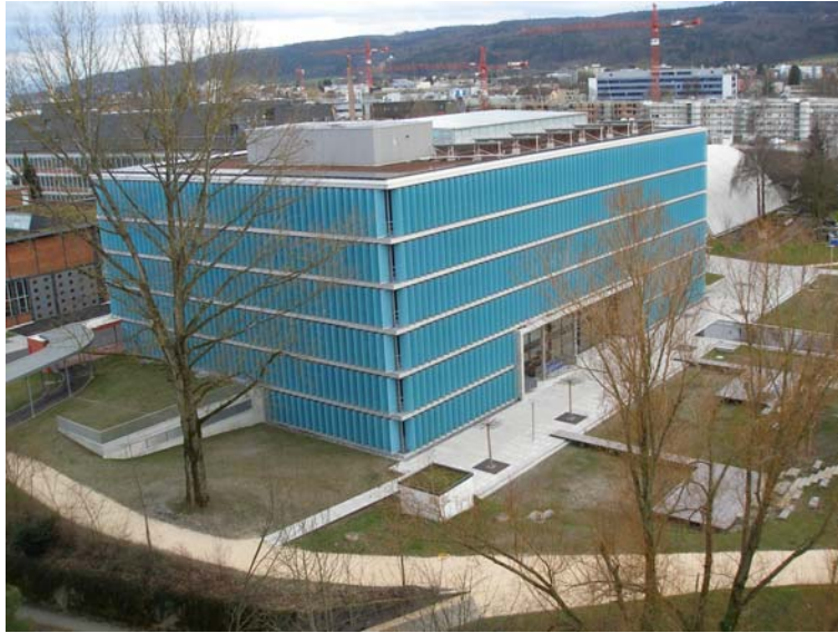
Figure 3 Eawag Forum Chriesbach: Characteristic facade with blue louvers, solar energy equipment on roof and air inlet of thermal register (behind tree on the NE - side of the building. Photo, A. Bryner Eawag 2. March 2007).
