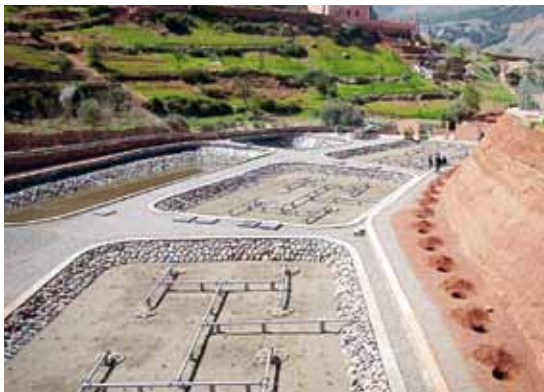
The new wastewater treatment facility serving a community of around 1,200 people south of Marrakech. Previously, wastewater flowed directly into the agricultural zone and the nearby river.
