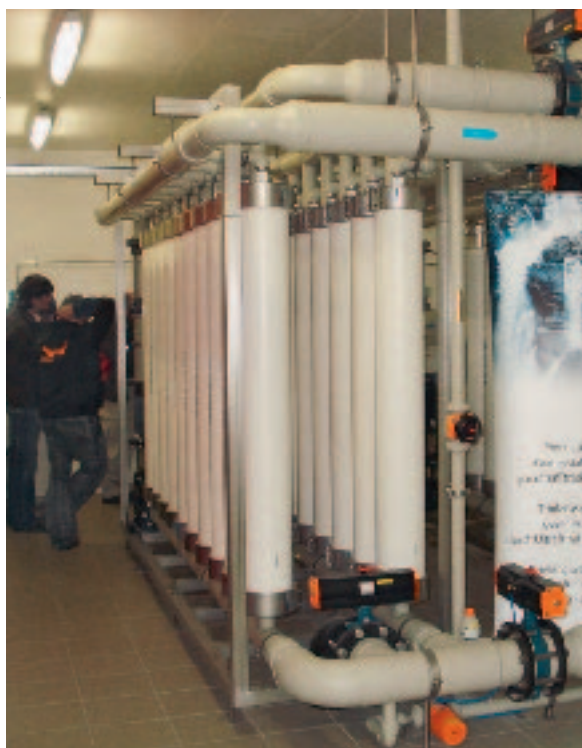
The ultrafiltration system in Frutigen (Canton Bern) comprises 40 modules (cylinders containing the membranes).
