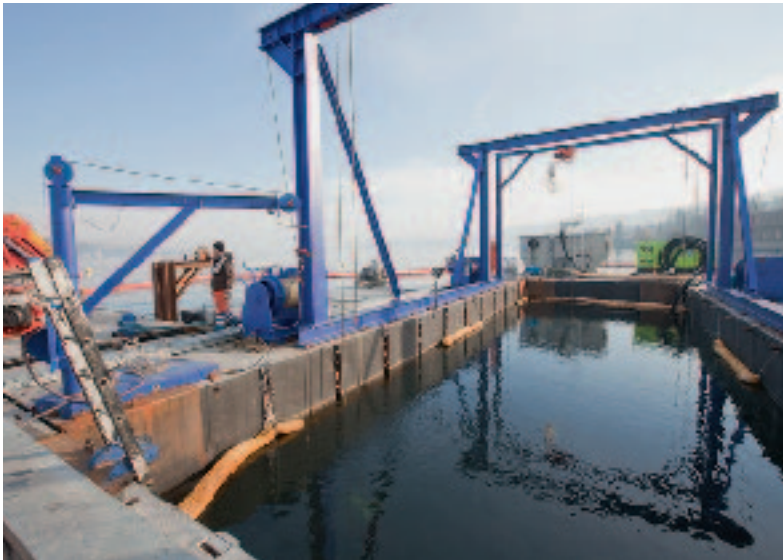
On the pontoon the sludge empties into a buffer tank and is then pumped ashore for treatment.
