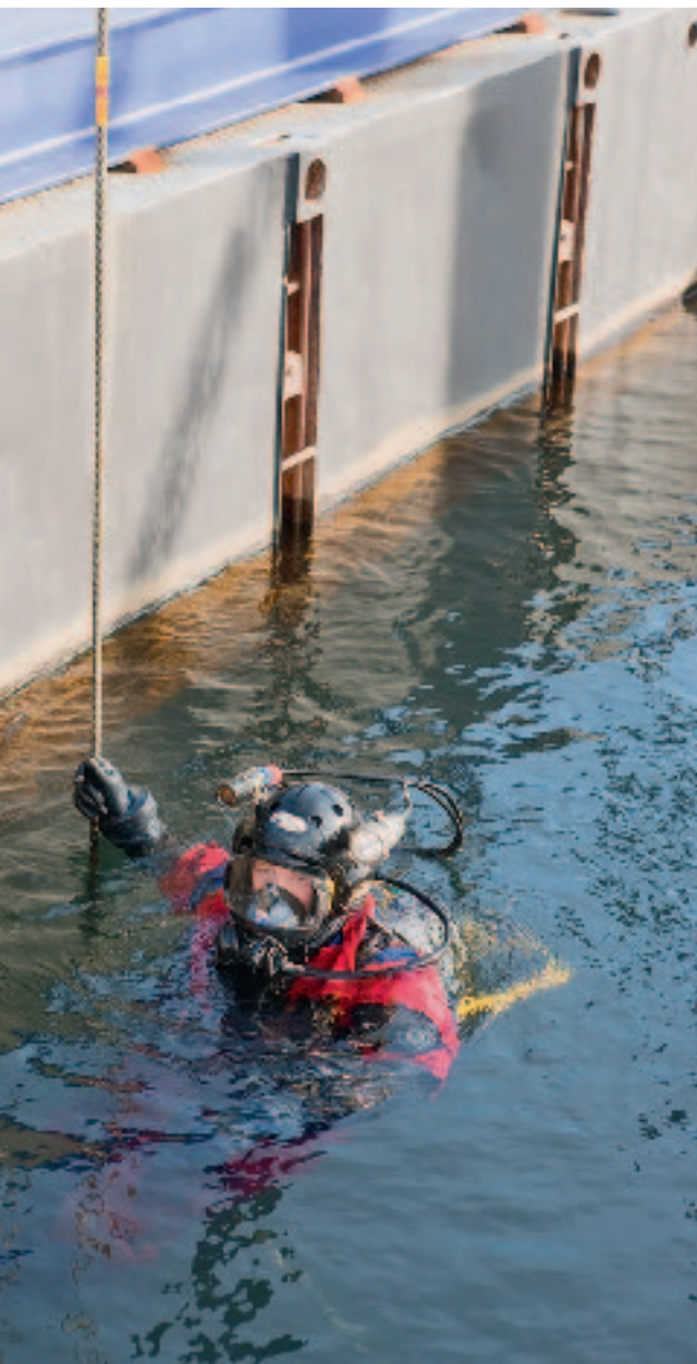
A diver can work on the lake bed (water temperature 5°C) for two hours at a time. His activities and the supply of an oxygen/nitrogen mixture are monitored by colleagues on the pontoon (small photo above).
