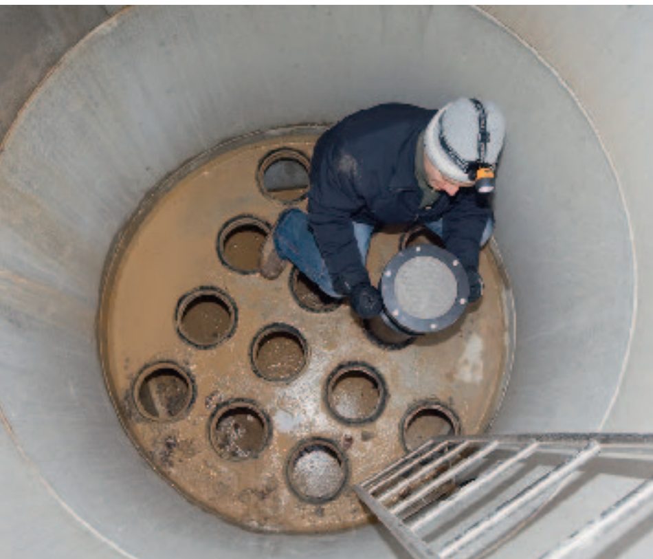
Filter cartridges containing granulated ferric hydroxide and calcite are inserted at the bottom of the drain.
