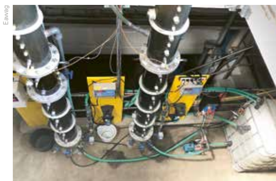
Pilot tests on GAC filtration at the Muri WWTP.
